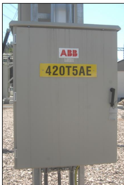
Figur 5: 420 kV effektbryter mot transformator T5, samleskinne A / Figure 5: 420 kV circuit breaker in connection with transformer T5, busbar A
